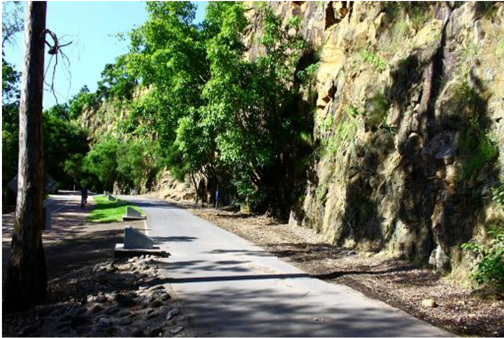
View of the cliff-line looking north from the access stairs
